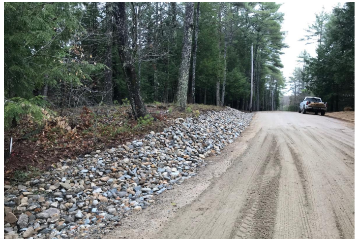
Before (left) and after (right) installation of riprap to stabilize embankment and capture sediment
