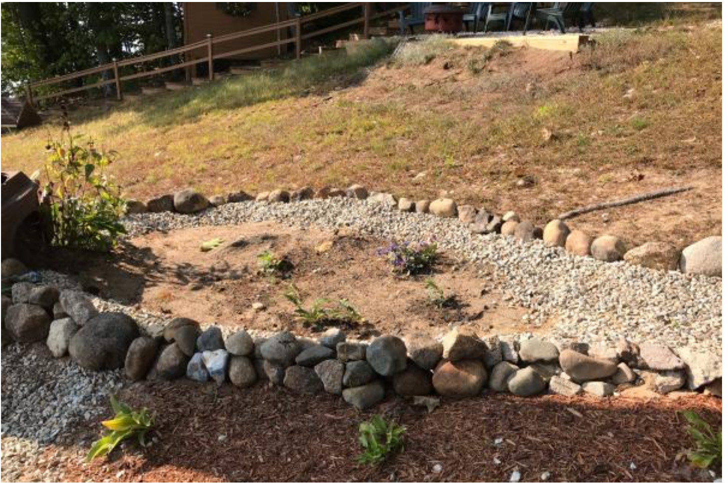
This rain garden creates a depression to capture and filter stormwater and grow beautiful native plants.
