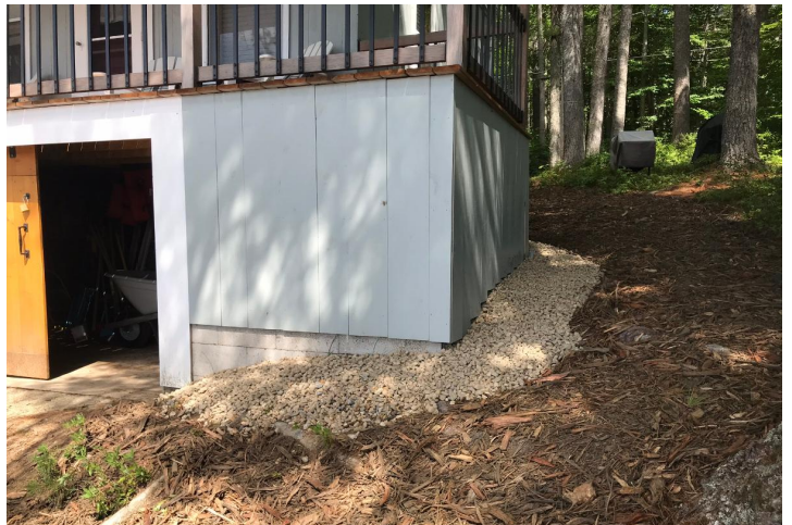
Before (left) and after (right) installation of conservation mulch and roof dripline infiltration trench
