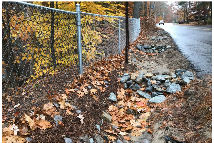
Before (left) and after (right) installation of stone check dams to capture sediment
